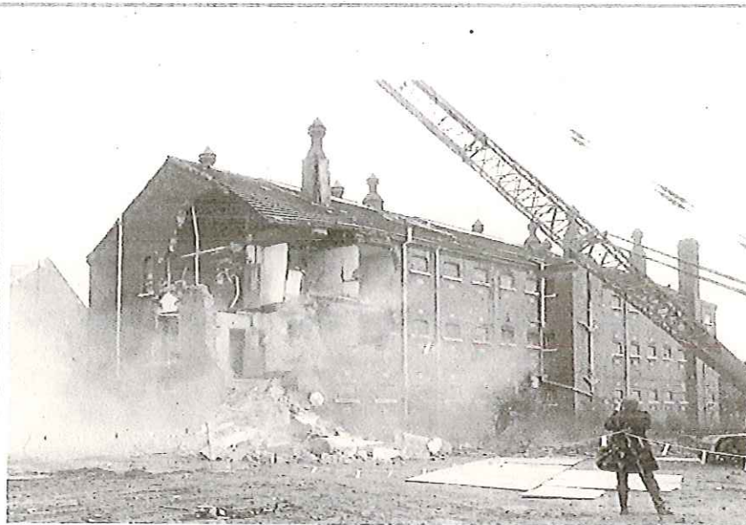
DX Wing shown being demolished in 1976.
